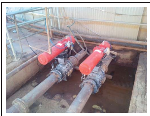
QuadroSphere® with Ring Master® Seating System for Geothermal Brine Clarifier Tank Valve
